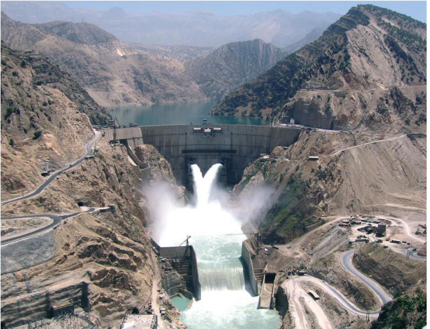
“Karun 3 dam with appurtenant hydraulic structures, spillway, outlet works, and stilling basin”, (Arch dam). 2004, Khuzestan Province, Iran, 205m in height”
