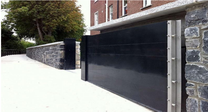
Fig. 1-2 FLOOD GATES BY RIVERS
