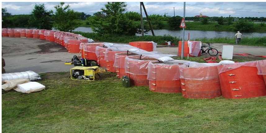
Fig. 1-3 For large scale flood defence, flood fighting and preparedness from river flooding, the Portable Cylinder Flood Barrier system provides a tried and tested alternative to sandbags.[2],[3],[4].
