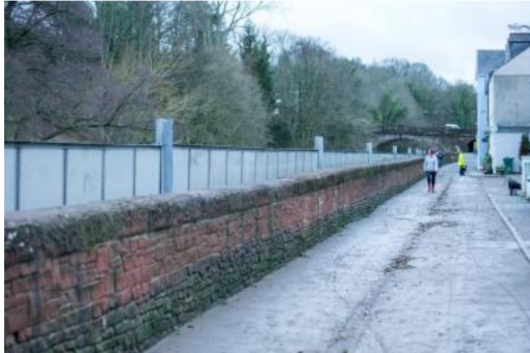
Fig. 1-4 Passive flood defence- Infrastructure Intelligence
